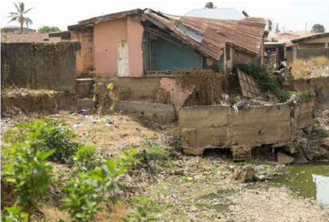
Flood ruins in Kabala West
